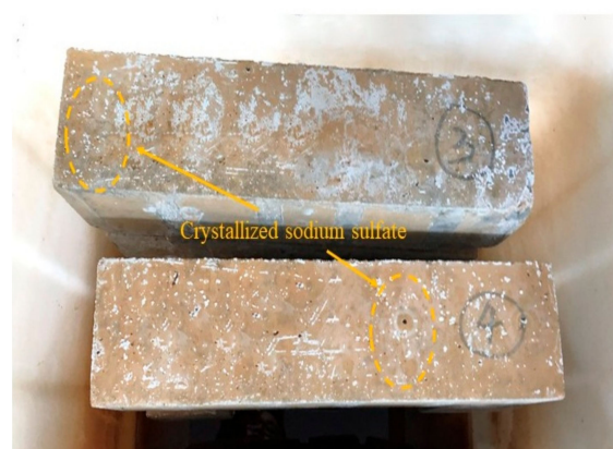
Figure 6. Crystallized sodium sulfate.
