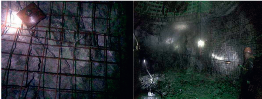
FIGURE 9: Effect of temporary on-site support.
